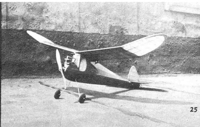
SINCE it was first introduced into model competition back in June 1944, the Kid has made quite a name for itself for consistency in winning high places in all the contests it has entered. It is easy to build, has enough strength to hold together but no excess construction to add weight. Above all, it possesses the ability to absorb all the power the motor is capable of producing.
