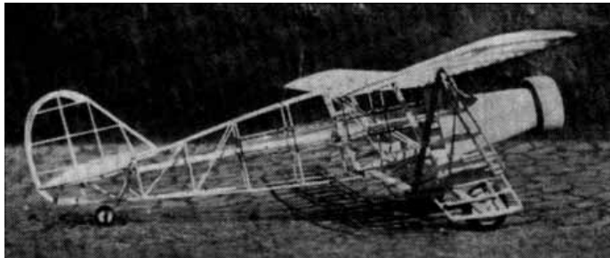
The completed uncovered framework indicates close adherence to the large plane design
